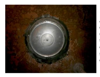
A flat fixing flange, a counter-flange to support the door, with a food-grade rubber gasket (interchangeable), and a door with assisted opening to facilitate centering and hermetic closing are installed on the internal wall of the tank, in AISI 304 stainless steel. The whole is sealed with waterproofing mortar certified for food use.
