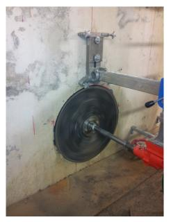
Access is achieved by drilling 800 cm of core into the tank wall. The through hole is drilled in a single solution using a special cutter.
